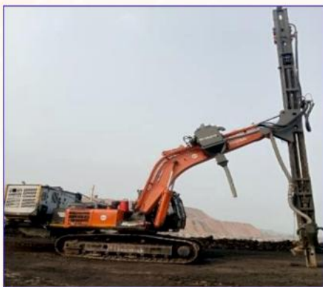
Drill Operation by Wet Drill Machines
