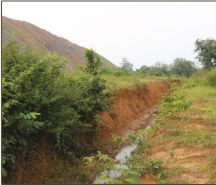
Garland drain provided around the OB dump
