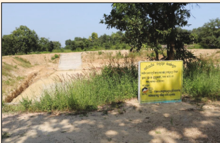
(Renovation of Pond with construction of bathing ghat at Village Kiripsira of Sanghumuda panchayat of Hemgir Block)
