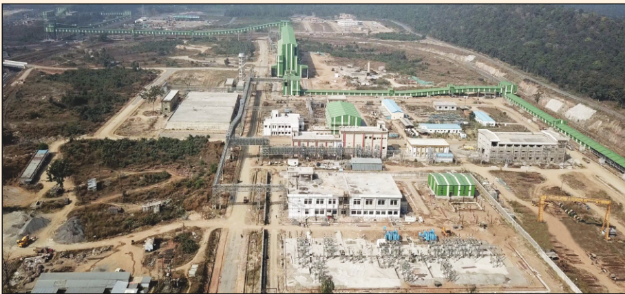
Coal Handling Plant
