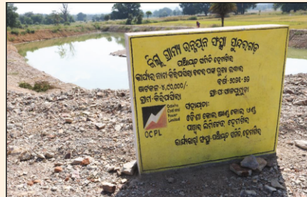
(Renovation of Pond with construction of bathing ghat at Village Durubaga of Durubaga panchayat of Hemgir Block.)
