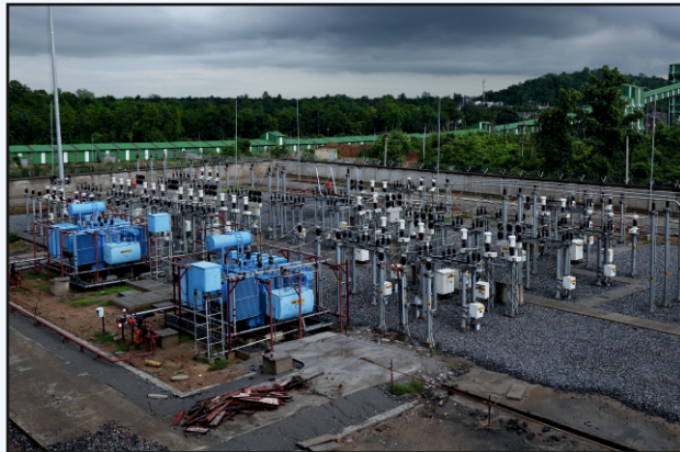
33/6.6 KV Substation & Switch Yard
